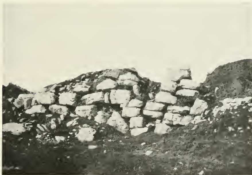
FIGURE 5. — A PIECE OF THE OUTER WALL ON THE WEST SIDE South of point 9
